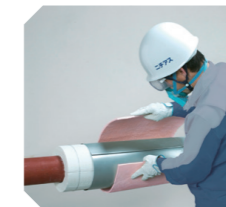
Heat retention maintenance work "Overlapped Heat Retention method"
