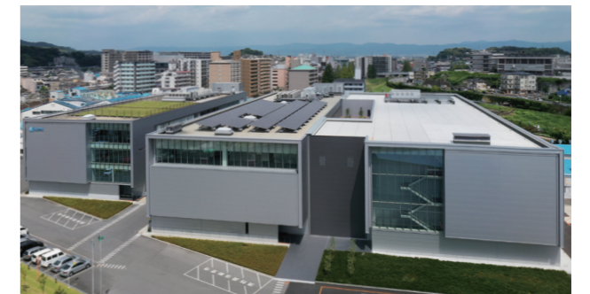
From left, New Building 1, New Building 2, New Building 3 of Ohji Factory (completed in June 2024)
