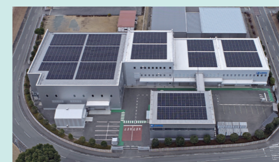
Solar-power-generation system facilities of Kumamoto NICHIAS
