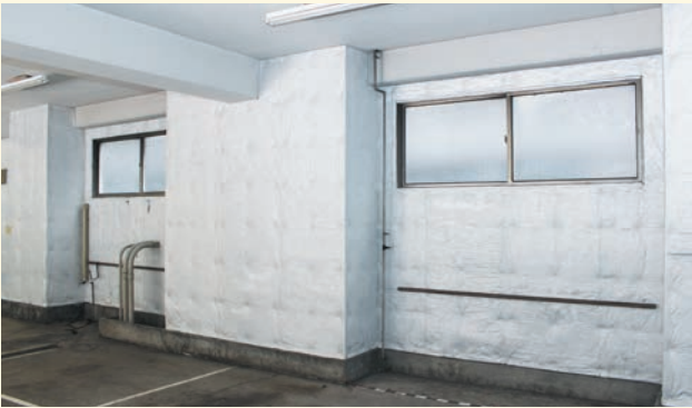
Car park : Heat & Sound insulation and Non-combustibility
