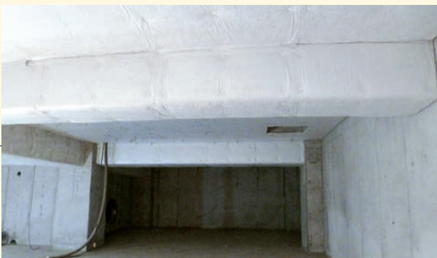
Pit : Non-combustibility and heat insulation
