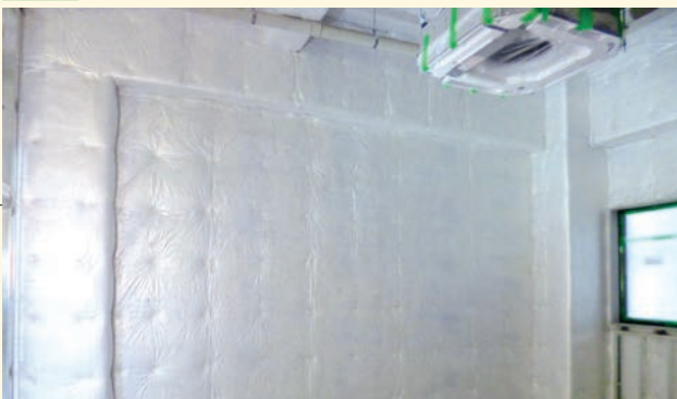
Wall : Out air attached heat insulation.
