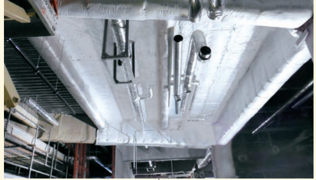
Ceiling Floor : Non-combustibility and heat insulation
