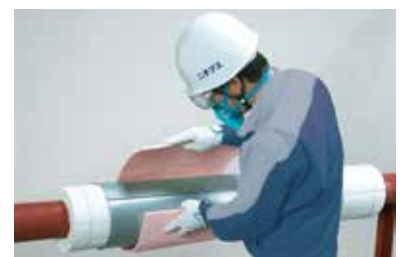
Overwrapping Insulation™ Method
