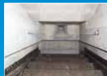
Sample of furnace lining work using castable refractory
